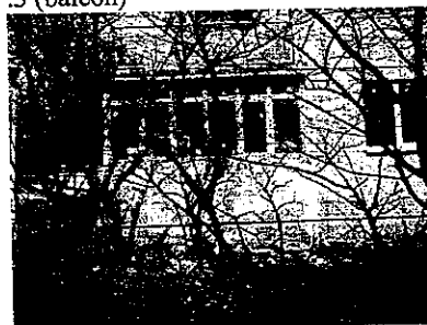
Teren = 3,75mp :bloc 47, parter ap 3 (balcon)
